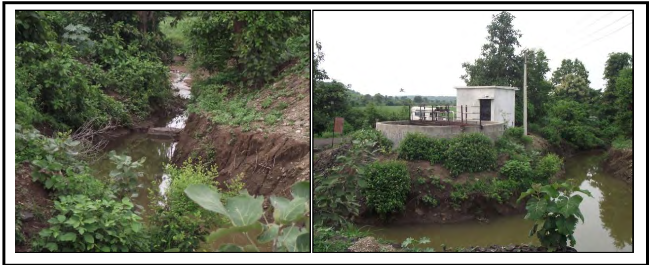
Fig 11.2: Recharge Shaft, PWS well and Under Ground Bundhara(UGB) (submerged in water) at Menkhat(Maharashtra)
